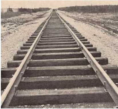
Fig 8 The Great Slave Railway - newly constructed in 1965
